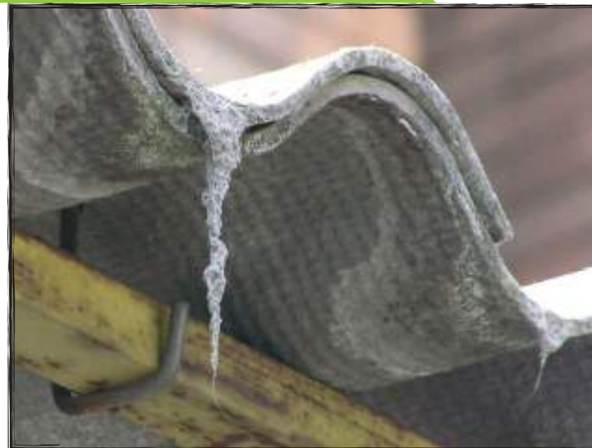
CHAPAS DE FIBROCEMENTO (ASBESTO-CEMENTO)
